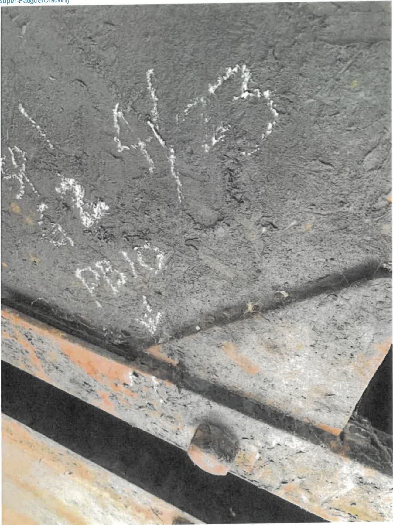
Photo #4 New crack in the weld connecting Angle 2 and Pontoon Box 10
